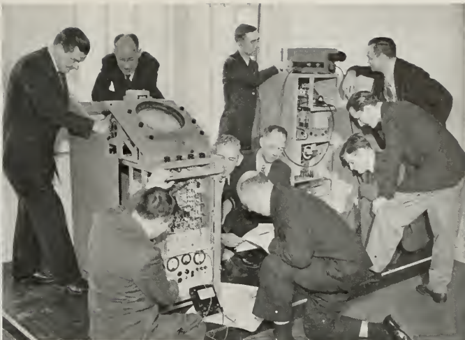
MEMBERS OF A CLASS AT RADIOMARINE STUDY METHODS OF SERVICING AND MAINTAINING MODERN RADAR UNITS FOR SHIPBOARD USE.
